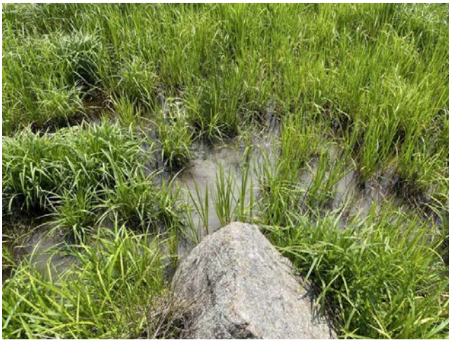
Photo 13: Facing down at existing conditions at Reach 02, June 3, 2025.
