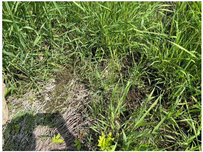
Photo 8: Facing down at existing conditions of Reach 1, June 3 2025.
